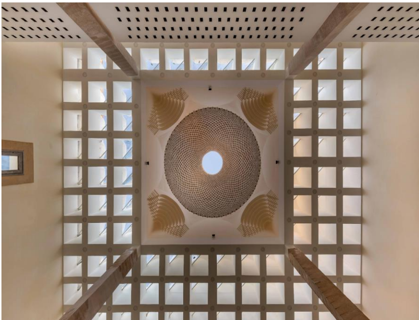
FIG. 3.15 An interior view of the central dome
