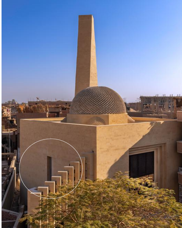
FIG. 3.16 An exterior facade showing the single window
