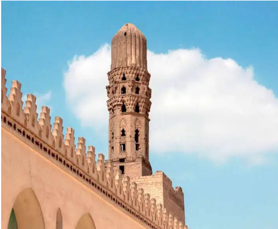
FIG. 2.5 One of the two minarets found in the two corners of main facade
